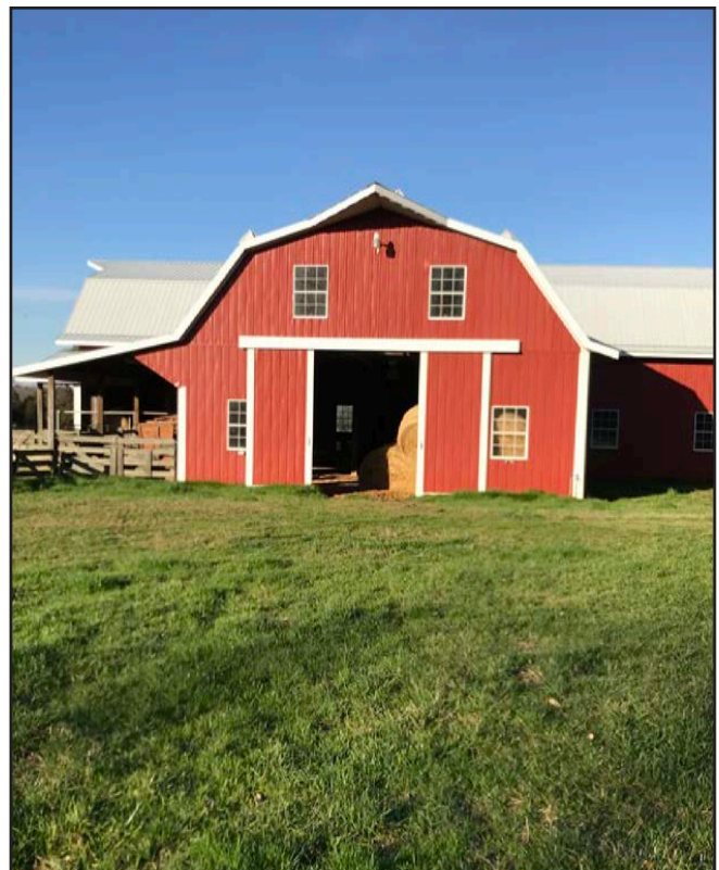
A barn in Southwest Alamance County
