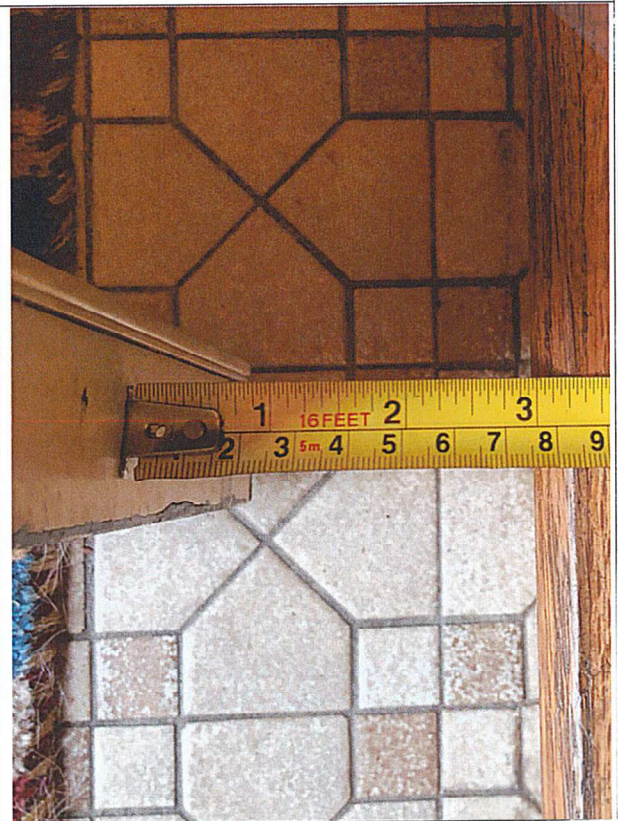
Figure 2 – Clearance between door and steps
