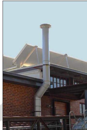
Figure 6: Industrial style vent pipe to match building exterior.
